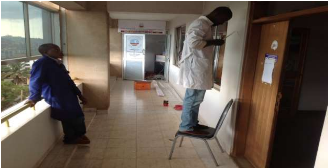
ELECTRICAL AND IT PERSONNEL WIRING THE OFFICE
